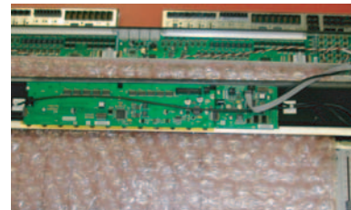
Step 6: Padding Material set on the Dual Fader Panels and the Meter Panel Removed
